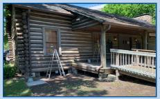
This is the eighth time the workers, using ladders, worked on the exterior surface of the logs in the restoration process—(1) wash, (2) hand sand, (3) & (4) brush on stain, (5) brush on matte finish, (6) repair chinking, (7) fill cracks in logs, (8) touch-up / final restoration
