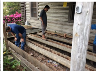
Front porch being rebuilt.
